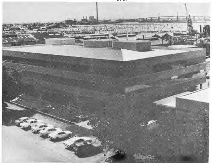
Nelson House, Williamstown Naval Dockyard administration offices.
