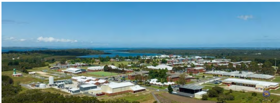
Aerial View of HMAS CERBERUS - December 2022 – much has changed as a result of the $600m redevelopment
